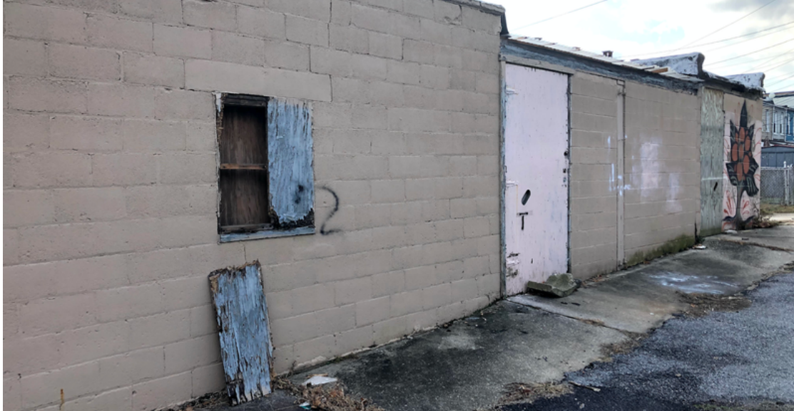
The alley BEFORE
